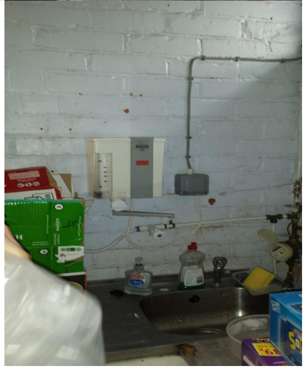
Picture on the left showing the entrance to the staff toilet blocked with stock. Picture on the top right showing more stock blocking access to the hand wash facilities. Bottom right shows additional hand wash facilities in the main store room. Again, obstructed by boxes of shop stock and also bags of rubbish. No soap in the hand soap dispenser and inadequate hot water facilities. Nowhere for staff to dry their hands.
